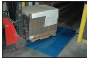
When in the parked position, the dock leveler is flush with the floor, eliminating concerns associated with trip hazard and cross-traffic obstructions.
